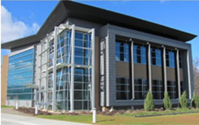
Stony Brook Advanced Energy Research and Technology Center
